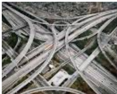
Figure 2. Road interchange in Nigeria.
